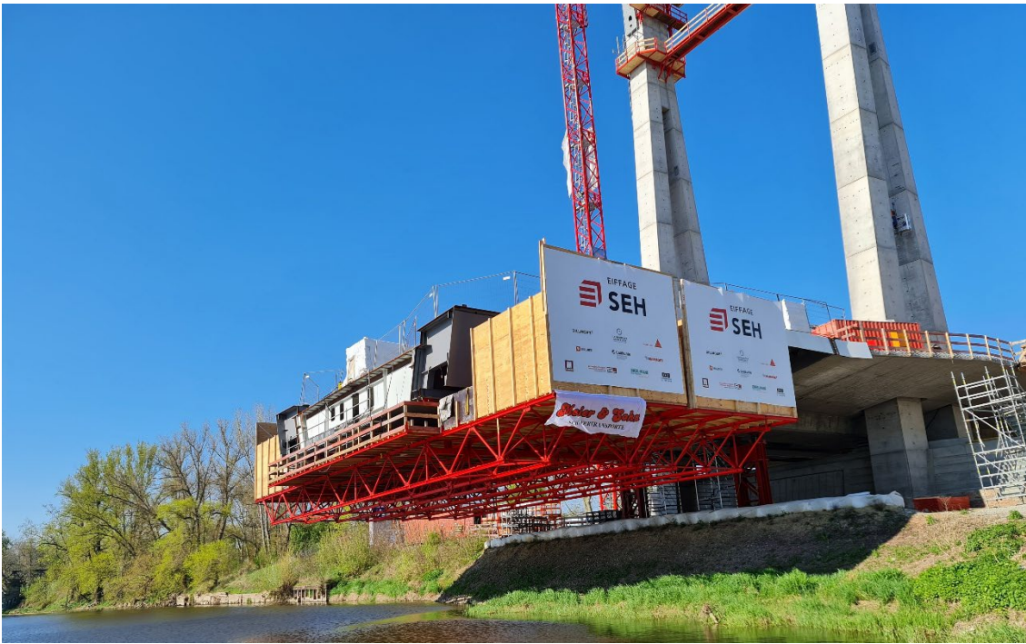
Figure 6: first shot installed under the use of combined welding and painting platforms
