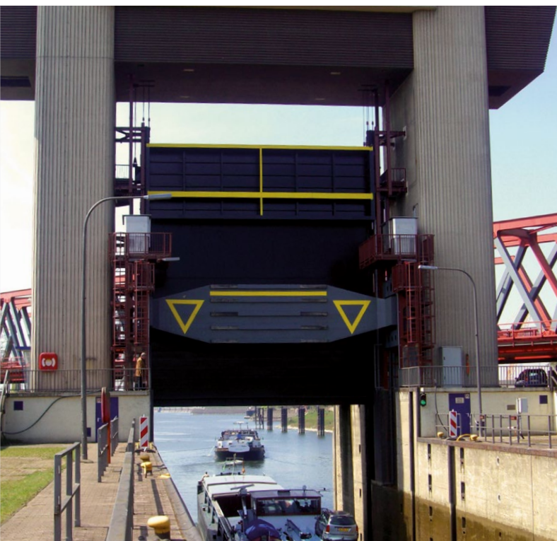
Lower gate 1 and 2 with buffer beams
