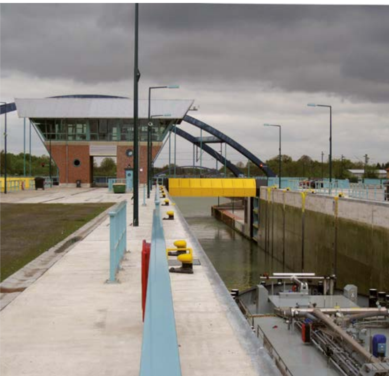
Buffering beam with lower gate
