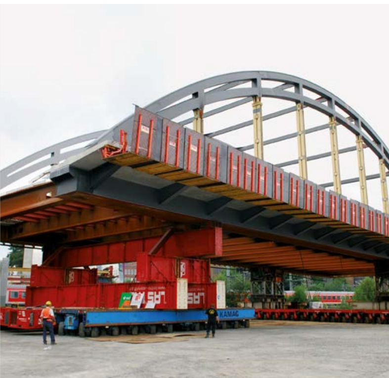
Erection of the arch bridge using SPMTs
