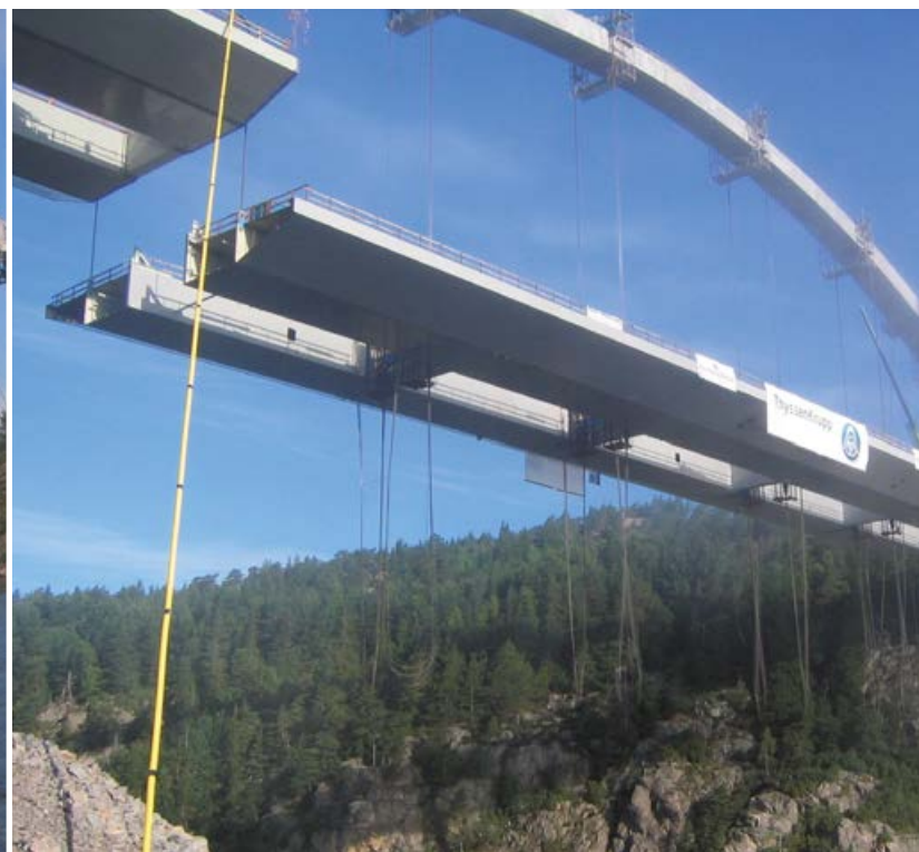
Lifting using strand jacks
