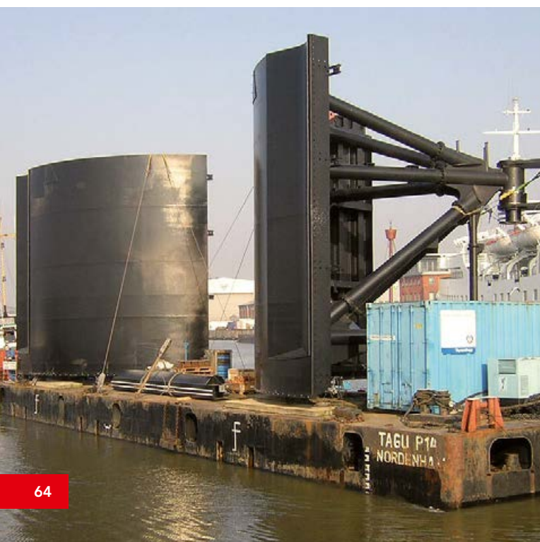
Transporting the two sector gates
