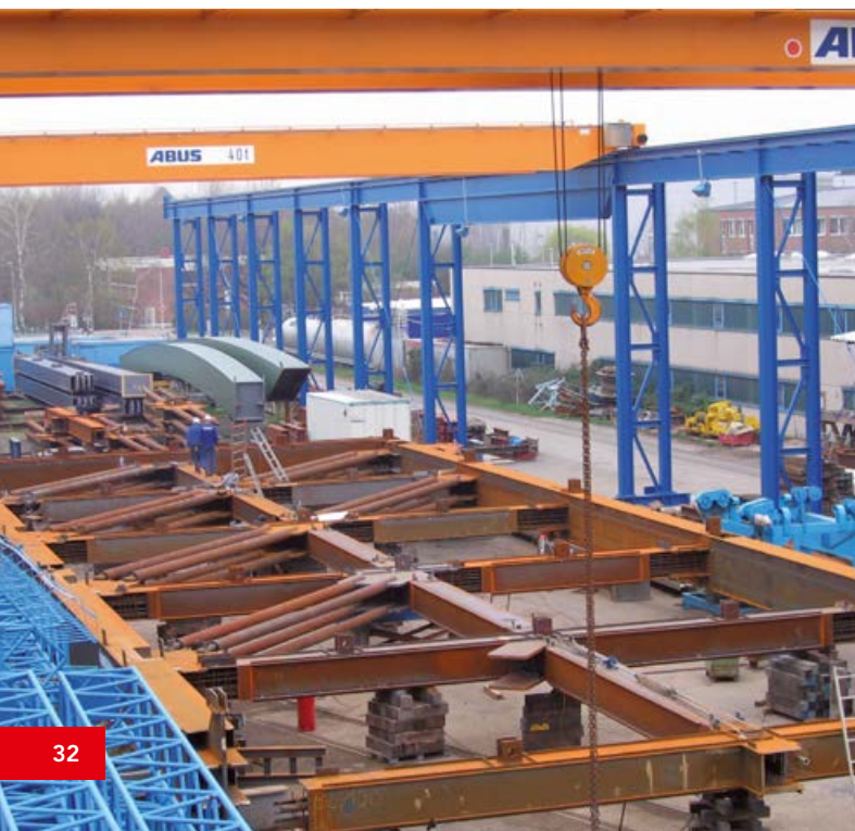
Preassembly of trusses in Hanover
