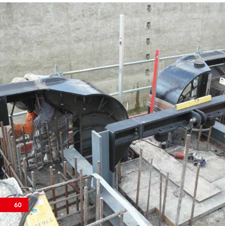
Adapter fitting at middle pier
