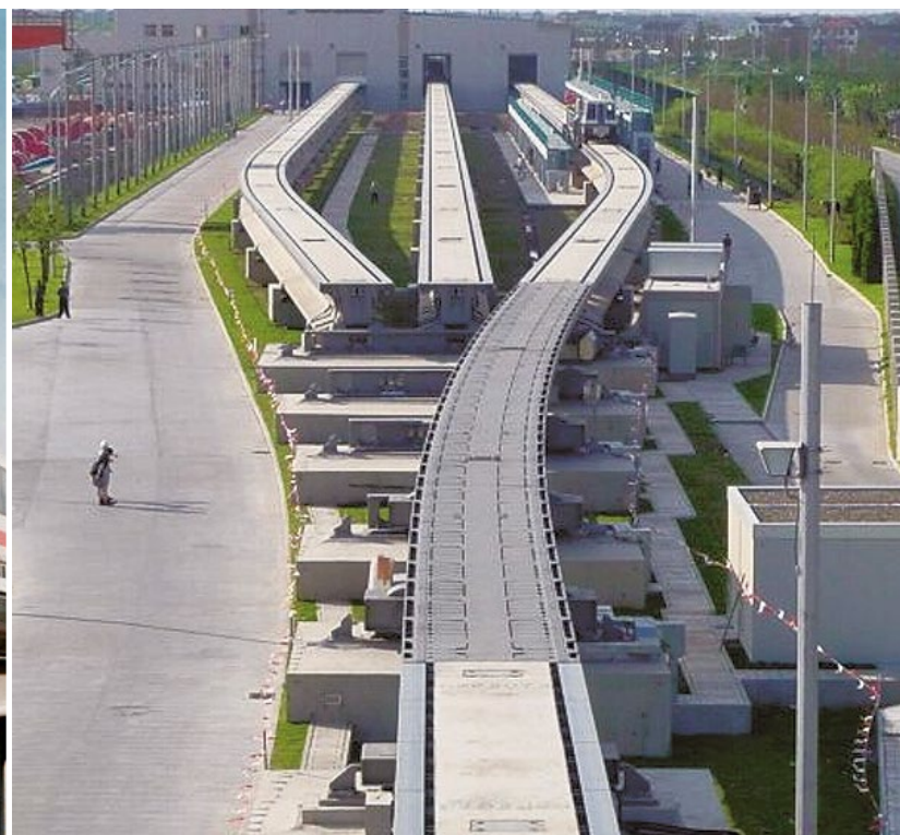
3-way movable track connection at the Shanghai Maintenance Center
