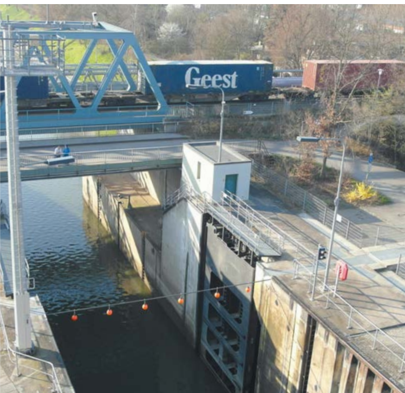
Sluice gate Feudenheim: Mitre gate at aft gate
