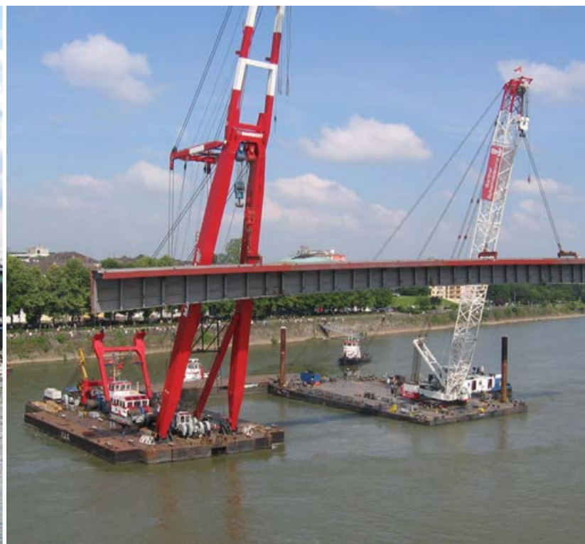
Erection using floating crane
