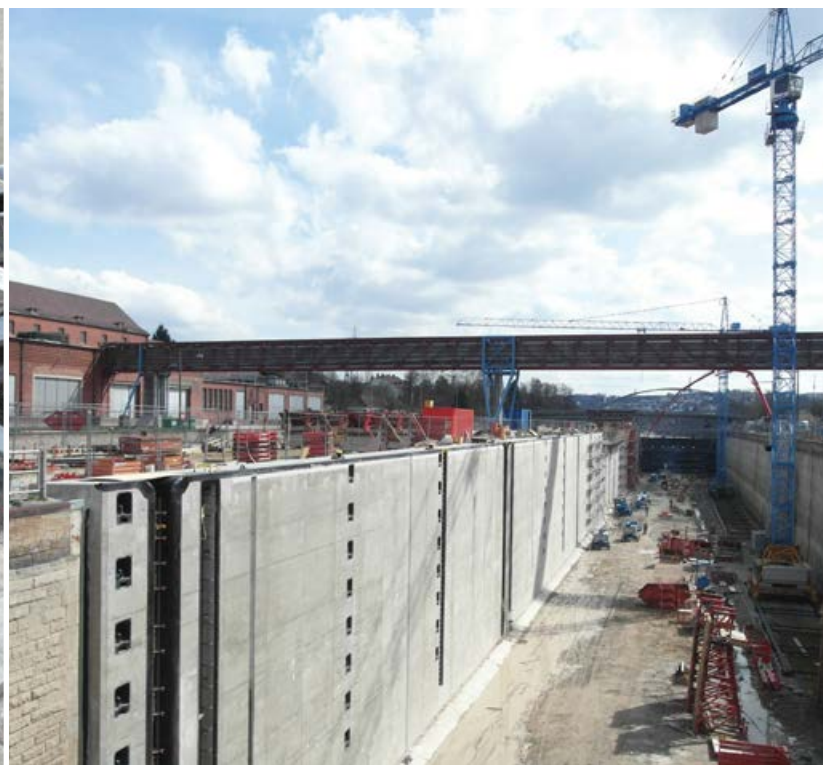
Guidance for floating bollards at middle pier
